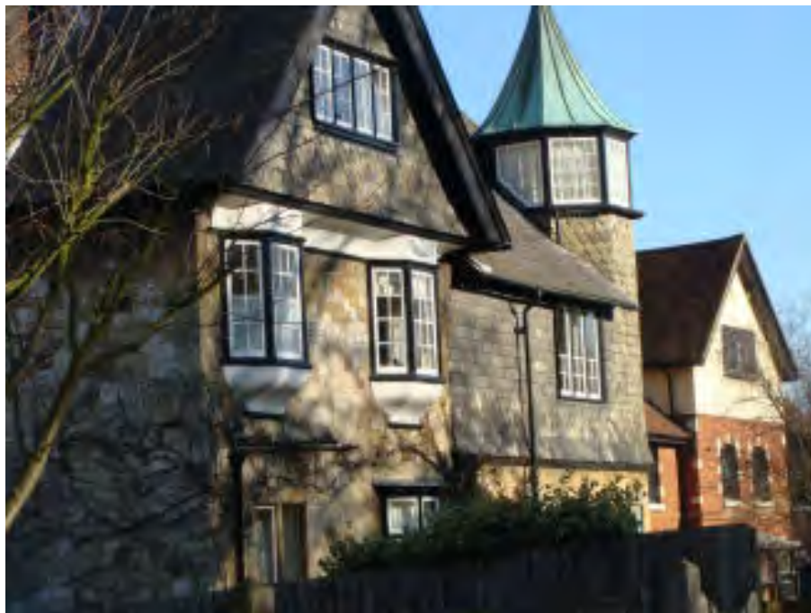
Picture 1.48 Nos. 9-10 Mount Pleasant Road, a fine 19th century listed building
