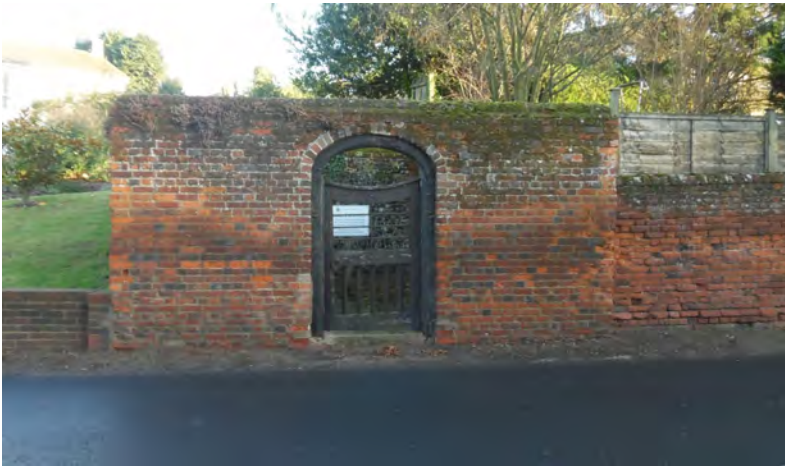
Picture 1.11 The Pound enclosure located on Little Walden Road, with brick elevations in English Bond and an opening with wooden door to the west elevation. There is a further blocked opening on the north elevation.
