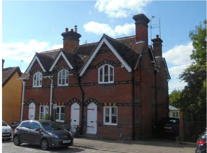
Picture 1.10 No's 77 - 81 Castle Street; a pleasing terrace of nineteenth century houses with prominent chimneys, elaborate decorative brickwork and patterned bargeboards.
