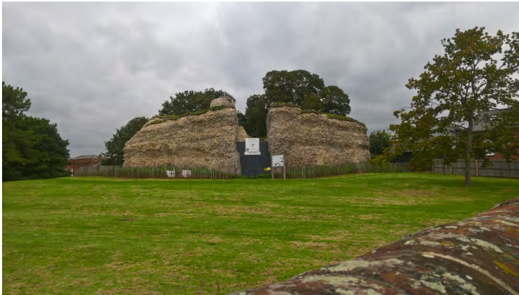
Picture 1.8 Saffron Walden Castle post soft capping works
