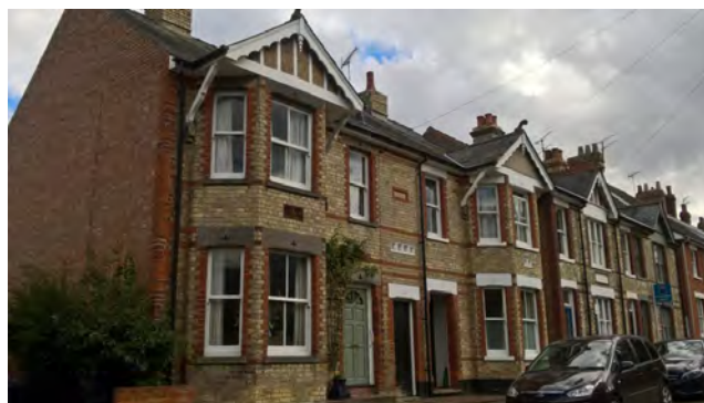
Picture 1.37 No.s 46 - 52 Fairycroft Road
